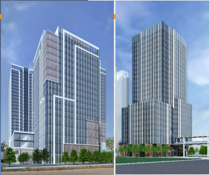
Nangang Business-Trade Park No.C2 and C4 Project
