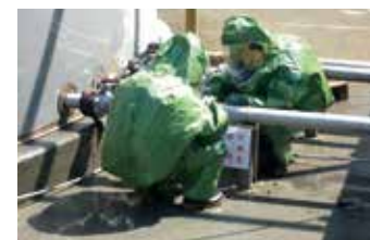
Emergency repairs of leaking pipes
