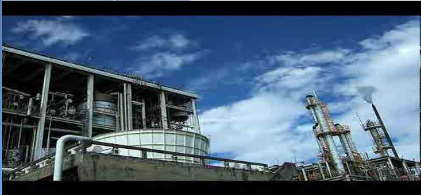
Taichung Relocation Plant
