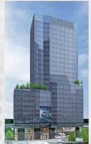
Nangang Business-Trade Park No.C4 Project
